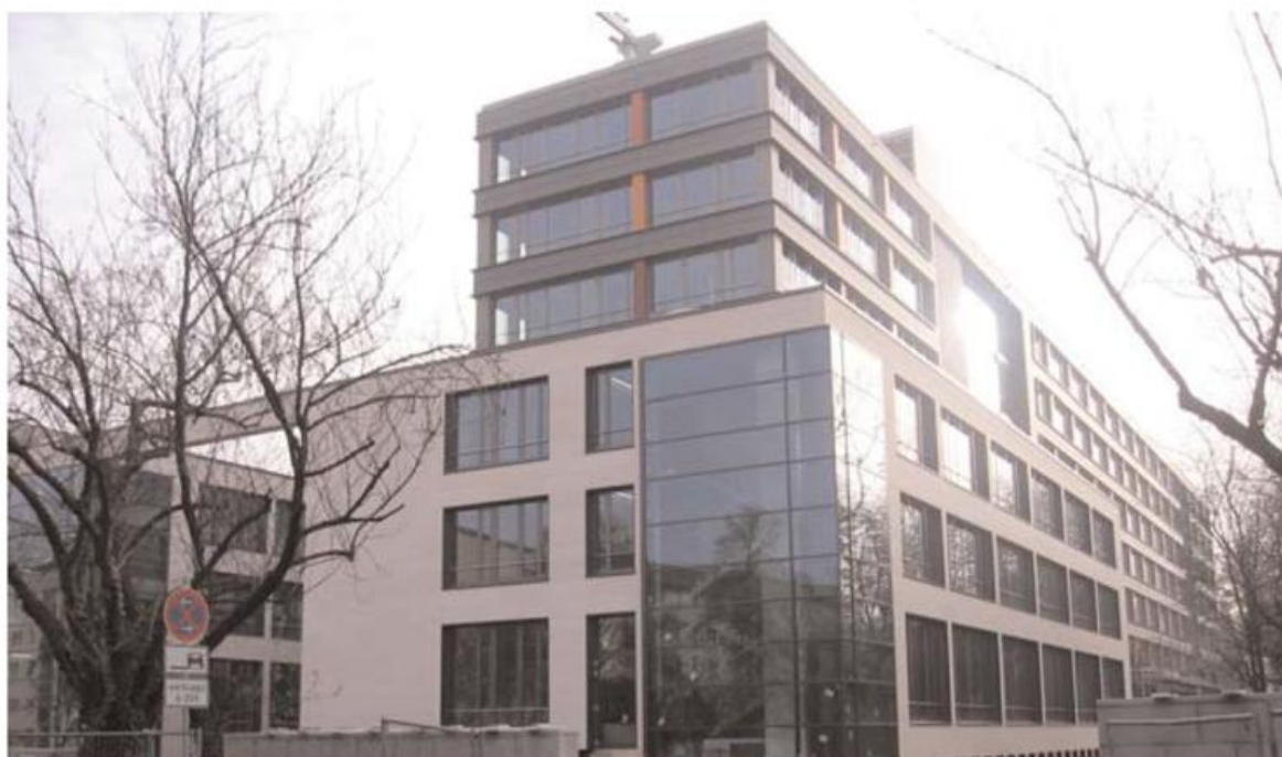
Der Neubau Anfang 2008 / New building at the beginning of 2008
