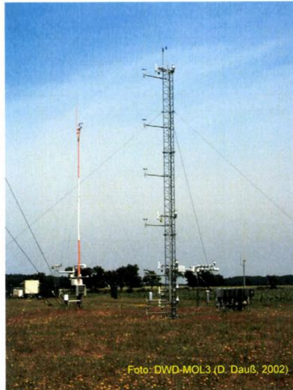
Figure 9 The 10 m mast for standard meteorological measurements from SSW
