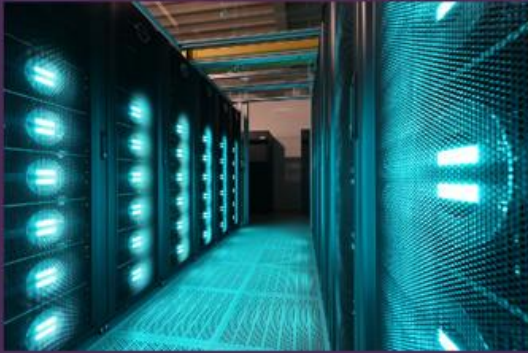
▲ Photo 5.4-2: View into the DKRZ's disk storage system
