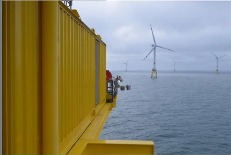
◀ Photo 3.5-2: At half of the measuring stations, redundant measurements are or were carried out using wave buoys or wave radars. In this offshore wind farm, the wave radar is fixed to the substation platform. Redundant measurements serve to compare the different measurement systems and improve data quality control methods.
