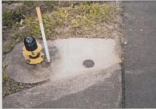
Figure 4: Water film sensor (dark round circular area). The sensor is located next to the paved surface. Sections of the grass-grown, concrete (grey) and tarmac (dark-grey) surfaces can be seen as well.
