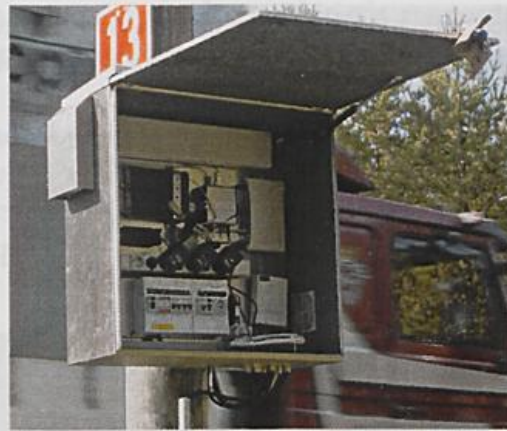
Picture 2. Device cabinet at roadside
